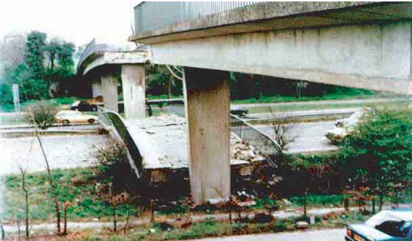
**PLATE 2 COLLAPSE OF A DECK SPAN FOLLOWING A COLLISION FROM AN EXCAVATOR TRANSPORTED ON A LOW LOADER
