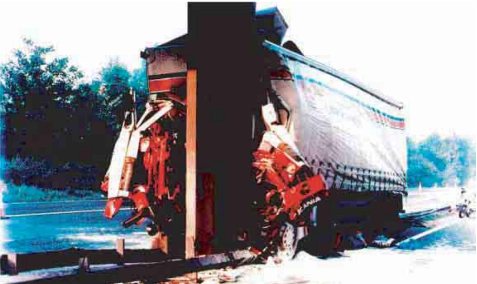
**PLATE 1 COLLISION OF HGV WITH REINFORCED CONCRETE SUPPORT M20 MOXLEY ROAD BRIDGE**
