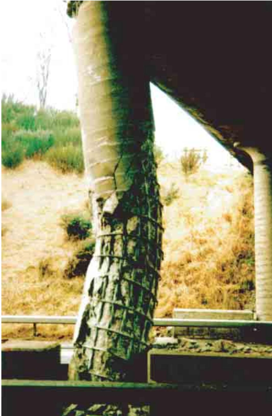
**PLATE 3 COLLISION DAMAGE TO REINFORCED CONCRETE CENTRAL SUPPORT
