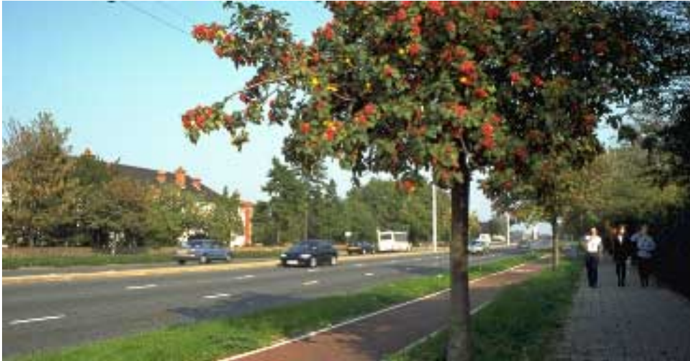
Great West Road The design and materials used for footways, boundaries and other infrastructure will play a key role in enhancing the amenity for residents and road users on the town approaches
