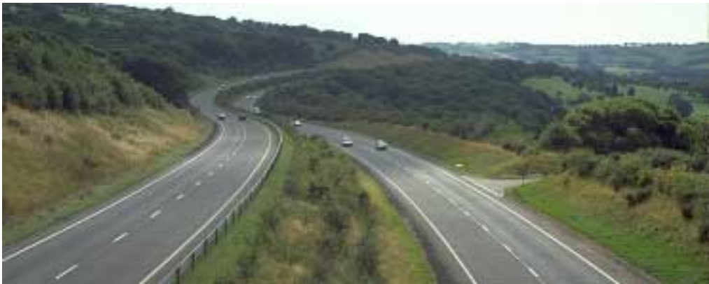
Okehampton Earthworks design is of primary importance for achieving a visually-acceptable corridor, particularly where planting to mask it would be inappropriate
