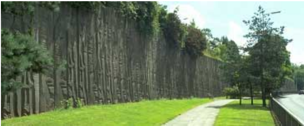
A451 Retaining Wall Relief Structural finishes can provide a dramatic feature and are set off by amenity grass within the public open space nearby
