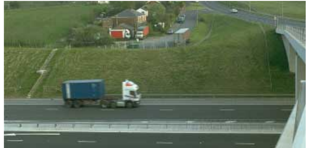
Noise Mound Noise mounds can be overbearing near housing and may need their form softening with planting. Species density choice and ultimate heights should be designed to reduce, rather than emphasise, the perceived height and mass of the mound
