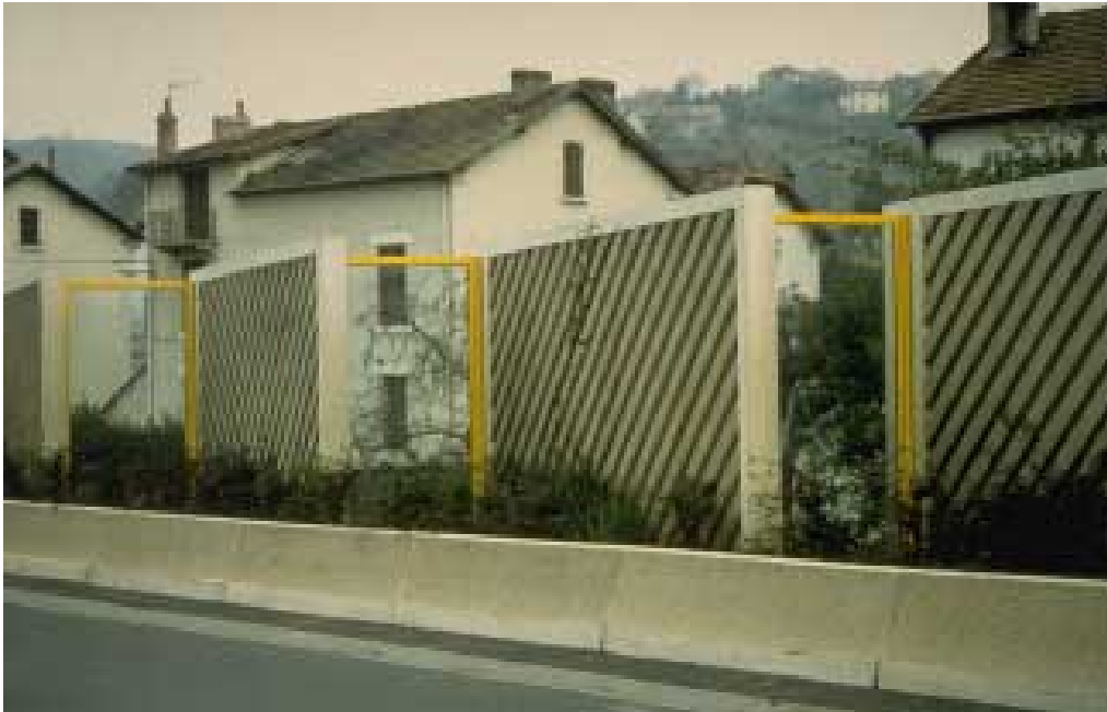
Noise Barrier The primary function of barriers is normally Noise or Visual Screening, but they should also be designed to provide Visual Amenity
