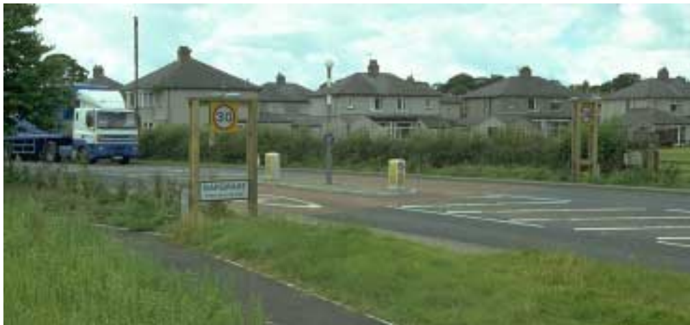
Gargrave Traffic Calming Safety schemes in villages need careful design to avoid intrusive features near residents' properties
