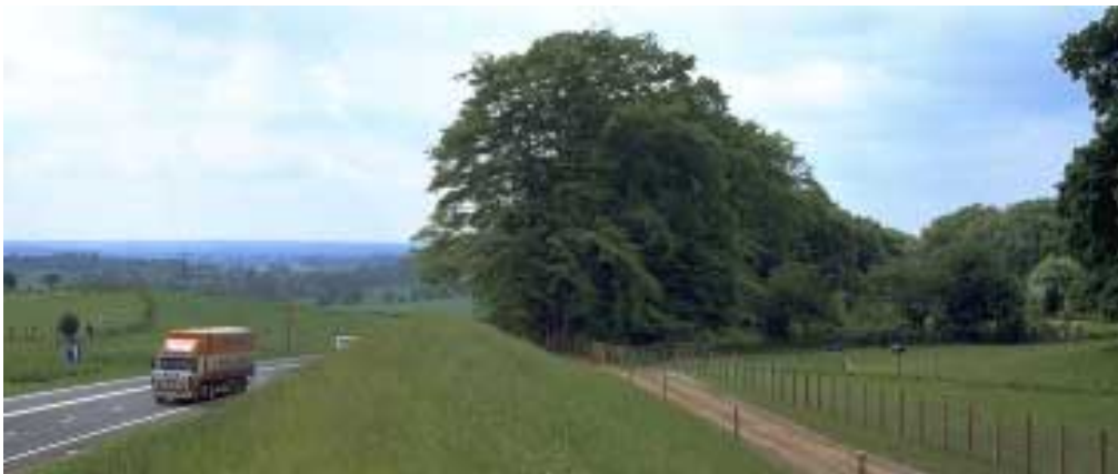
Earthwork Screen Earthworks used as a screen where linear planting would unnecessarily cut off views of the surrounding landscape
