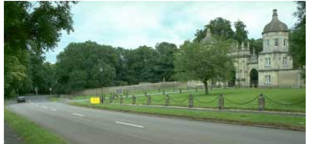
Burghley House Gates Maintenance standards need to reflect and integrate those used on adjacent properties
