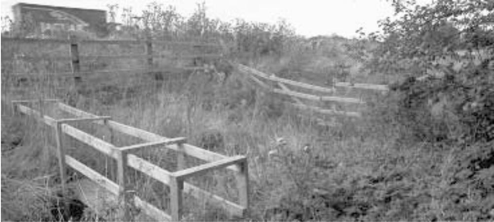
**Badger tunnel** *This structure extends the badger tunnel protection over the highway drainage ditch to safer habitat, alerting maintenance operators to the Element’*
