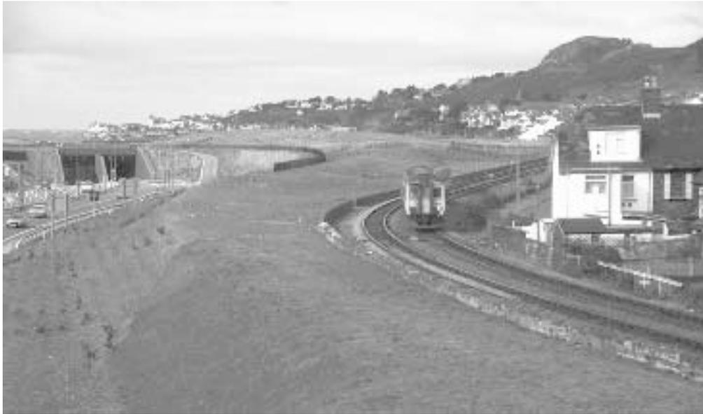
**A55 Conwy tunnel approach** *Deep cutting combined with raised mounding attenuates noise levels for adjacent properties*
