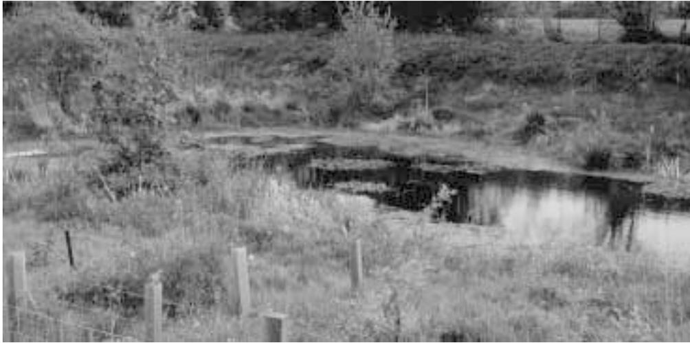
**Balancing pond** *Balancing pond for stormwater control and filtration*
