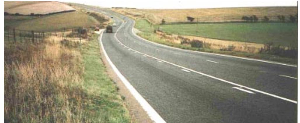
*Integration is largely a matter of good route alignment to fit the topography and the avoidance of roadside planting or conspicuous fencing which emphasise the line of the road. Grading out of earthworks and restoration to agriculture must always be considered.*
