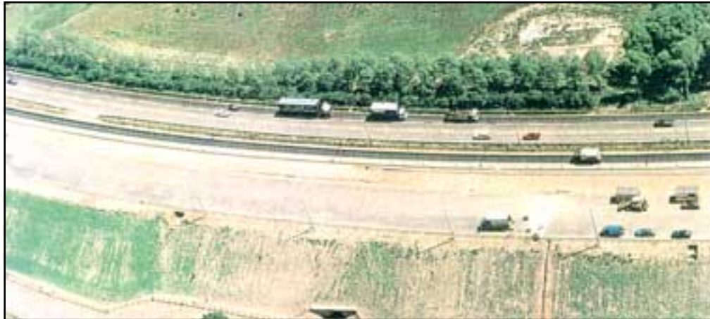
M5, between Lydiate Ash and Catshill. Asymmetric widening has allowed the retention of mature planting on the unwidened side to protect nearby housing.
