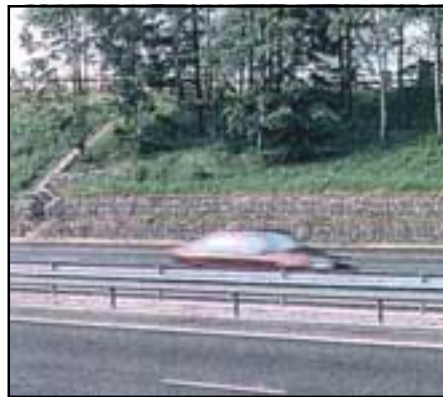
M40 Stockenchuch, gabions offer a flexible method of saving mature vegetation.
