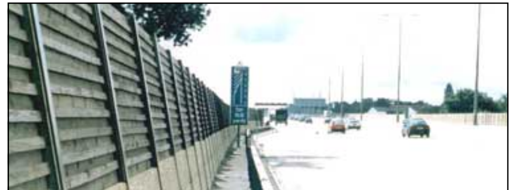
The reduction of unnecessary structure. There may be scope to select the type of safety fence and method of support. In some cases steel safety fences can be supported by the retaining wall and in others it may be possible to design the wall itself as a vertical barrier.
