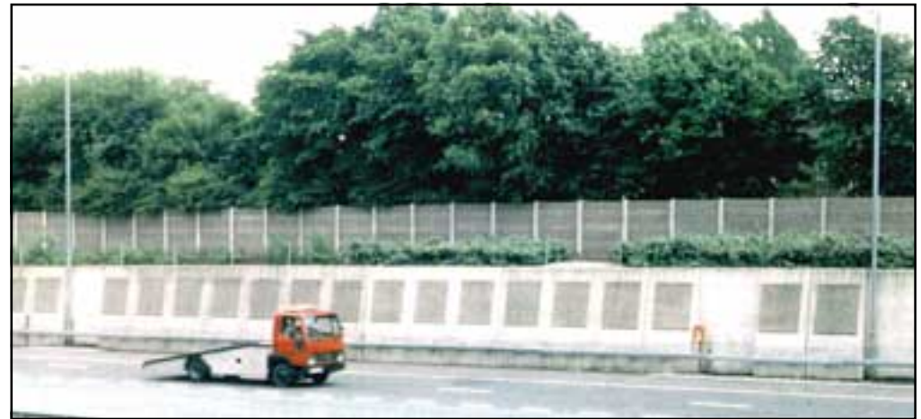
M56 south of Manchester. Symmetrical widening within the highway boundary through the use of the retaining walls has facilitated the retention of mature woodland planting and protected nearby housing.
