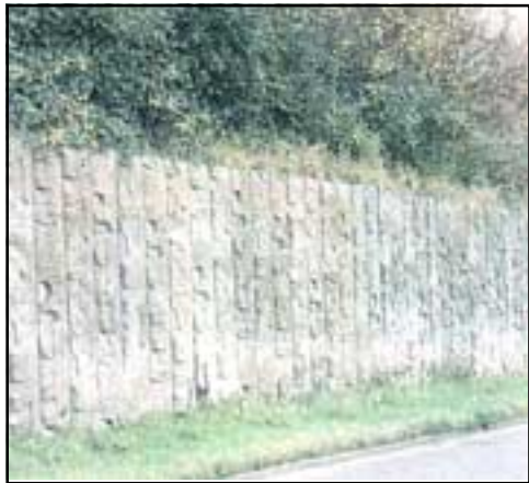
Coarse textured panels can be used to break up the visual mass of a wall.
