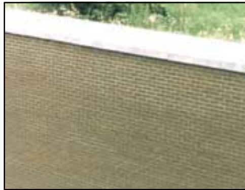
Brick or concrete precast units can be used to face insitu concrete retaining walls. This allows the use of more intricate designs and better quality control.
