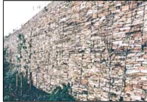
Gabions with coursed stone facing
