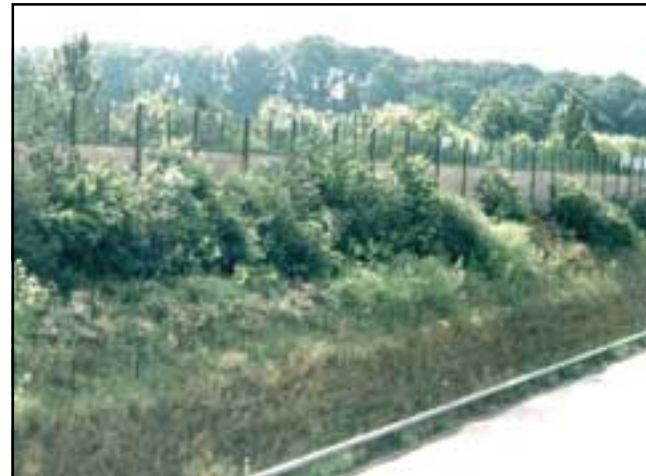
M25, Junction 10-11. Symmetrical widening within the existing highway boundary through the use of reinforced earth banks has allowed the retention of much of the original mitigation planting. This planting has a fundamental role in reducing the visual impact of a 5 metre environmental barrier.
