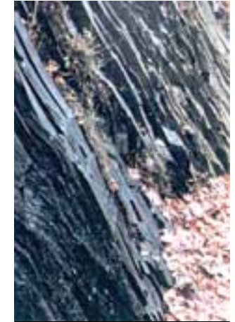
Well defined vertical fissures
