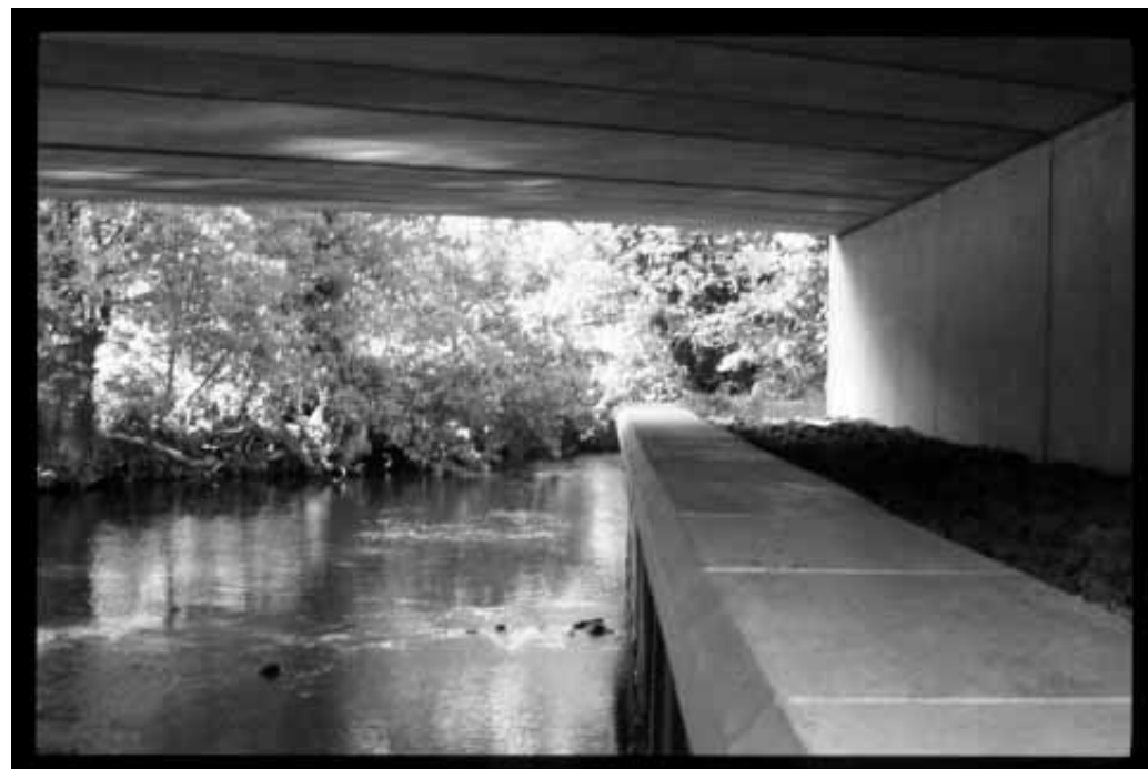
Hole Bridge, Bovey Tracey, Devon. A ledge was incorporated into the bridge design during construction.
