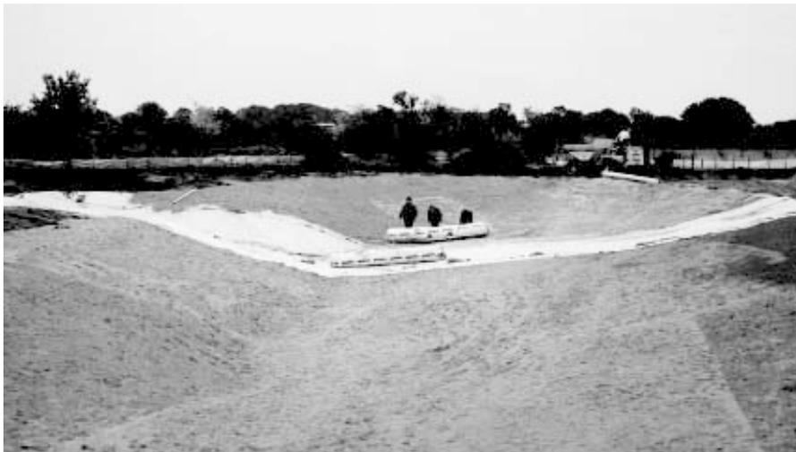
**Plate 4** *Lining large waterbodies requires detailed design and installation with natural materials to protect and disguise them*
