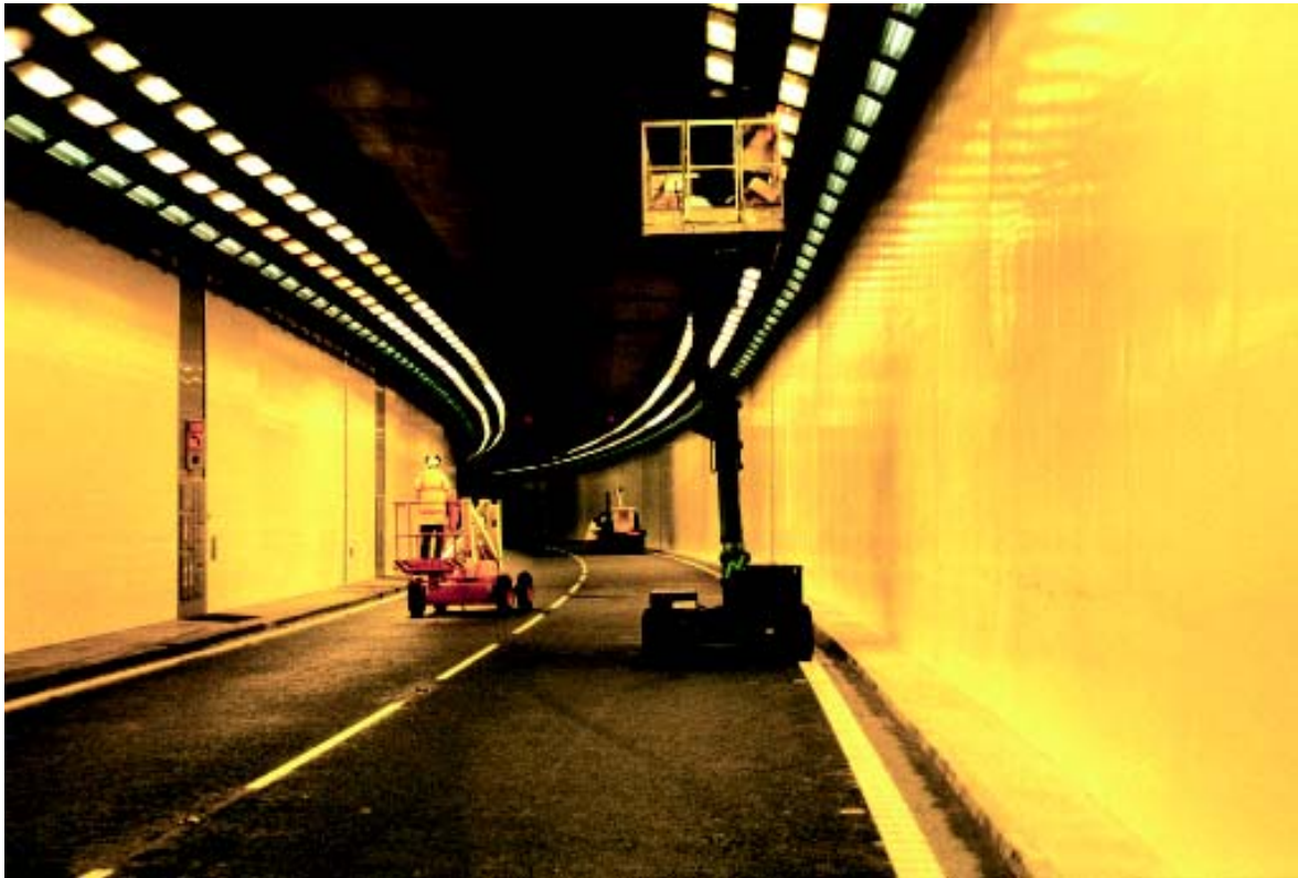
Figure 8. 1: Cleaning the Luminaires
