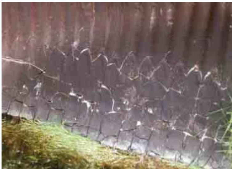
Figure B.6 Use of liner plates to protect an invert
