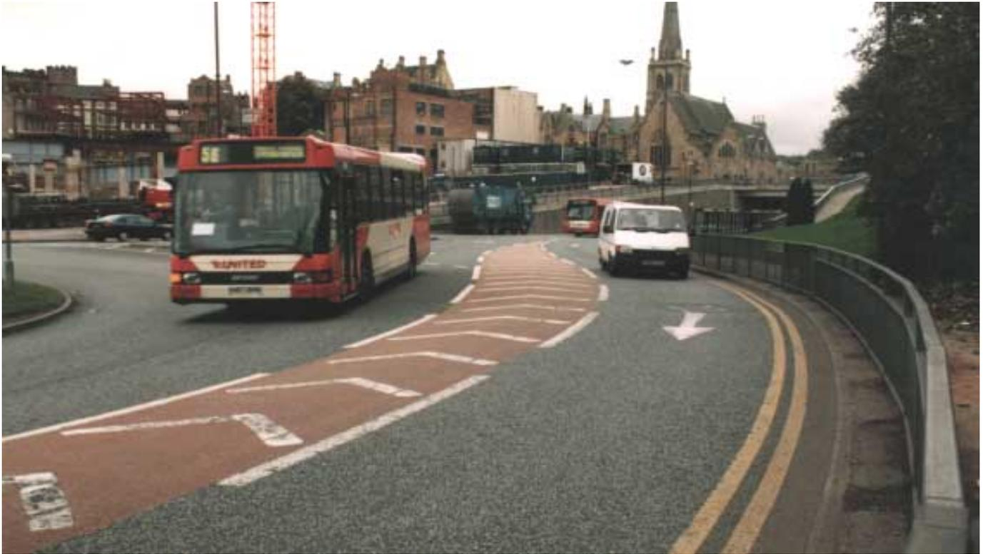
**Plate 5 Coloured Surfacing used to Improve Contrast on a Segregated Left Turn Lane at a Roundabout**
