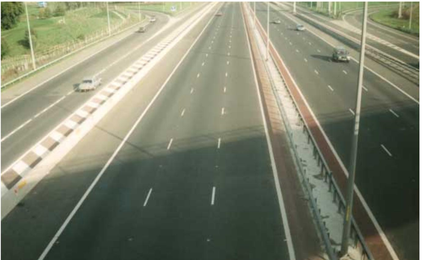
**Plate 4 Coloured Surfacing used to Improve Contrast Along Margins to Deter Over-Running**
