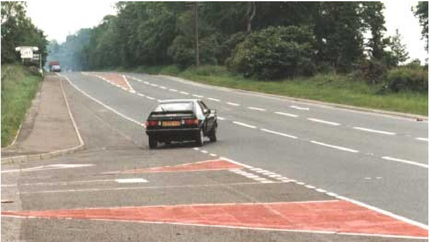
**Plate 6 Coloured Surfacing used to Improve Contrast in the Island Area of Priority Junction**
