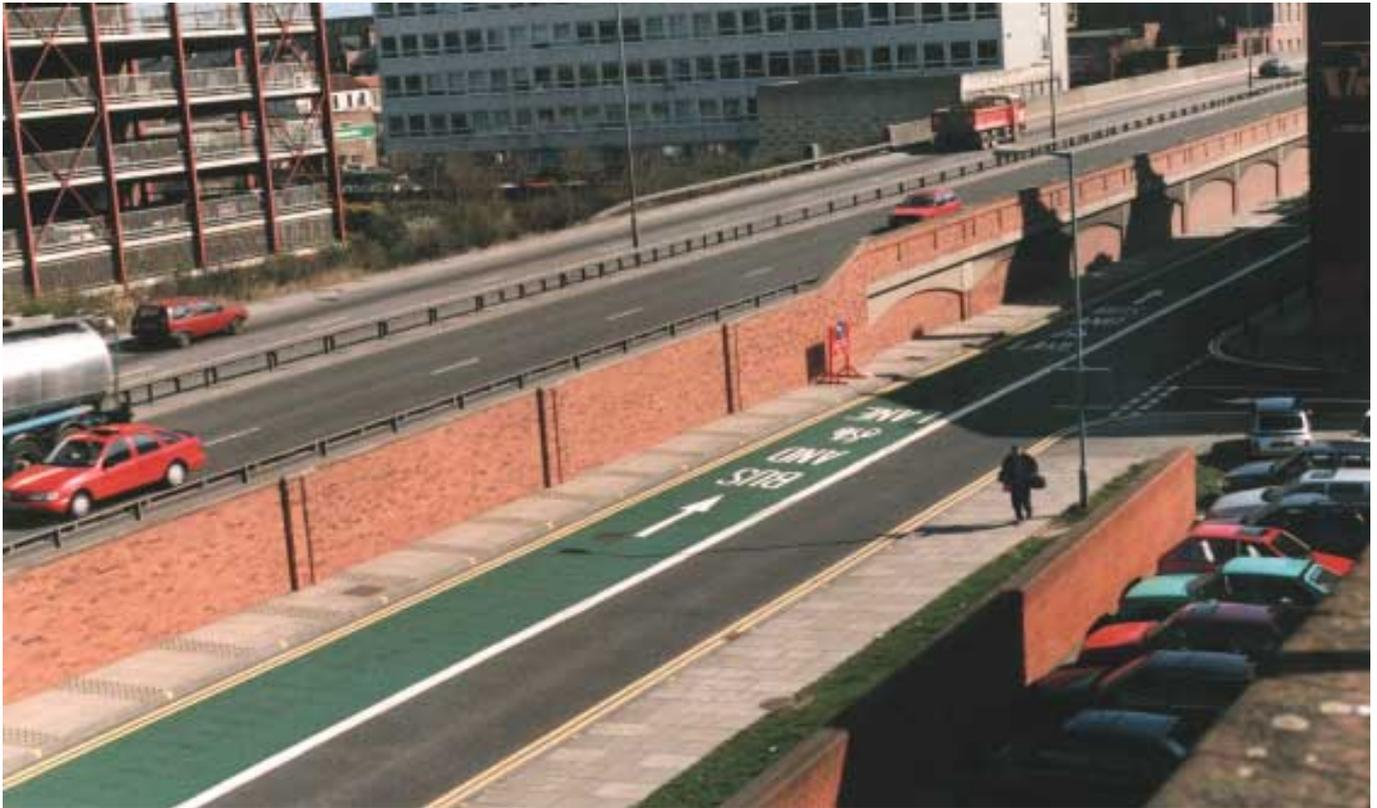
Plate 7 Coloured Surfacing used to Supplement Road Markings on a “Contraflow” Bus and Cycle Lane
