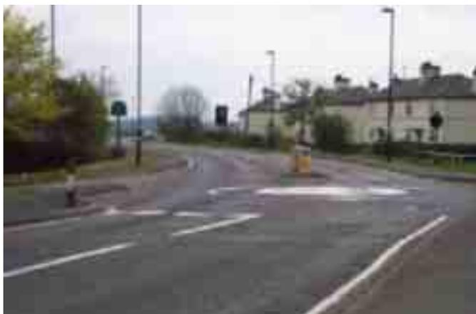
3.33 Mini roundabouts can be used within settlements, usually on roads of 30mph or less, as a means of slowing traffic. They can also substantially reduce accidents. However, it is necessary to ensure that the flows on the various arms feeding into the roundabout are reasonably balanced so that there are no unacceptable delays to main road traffic but that side road flows are sufficient to ensure that main road traffic does have to slow down.
