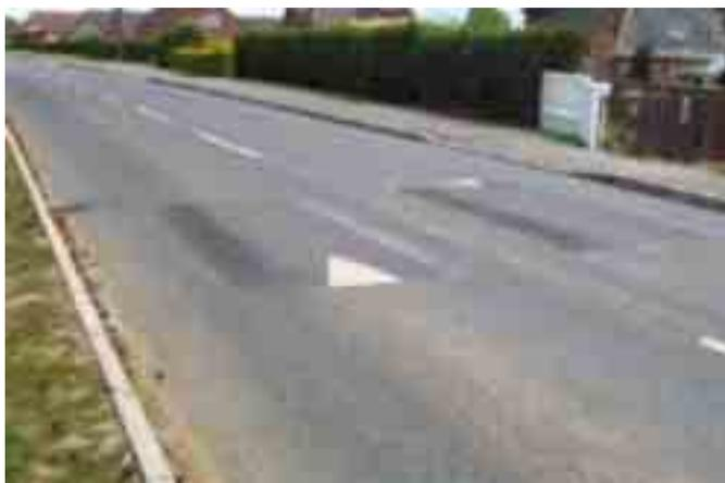
3.49 Whilst the opportunities on the trunk road network for using measures involving vertical deflection are limited, speed cushions can be appropriate. Cushions are a form of hump that are
