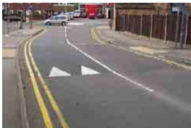
3.51 On trunk roads where there are relatively large traffic flows and high proportions of large vehicles, road humps are unlikely to be used. Nevertheless, at locations where they are considered appropriate it is important that they comply fully with current regulations, including signing and markings. It should be noted that road humps cannot be installed on roads with speed limits greater than 30mph without special authorisation.
