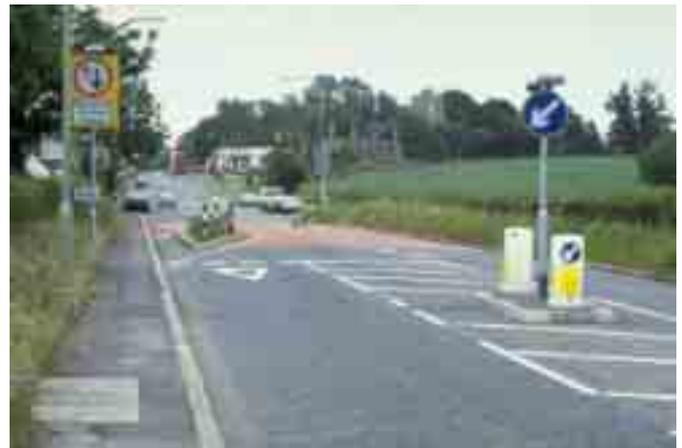
3.35 Single chicanes can reduce speeds by up to 20mph. However, chicanes designed to reduce car speeds down to about 20mph will be too tight for articulated HGVs. Designs to allow buses, coaches and articulated HGVs to pass through at 20mph will have little effect on cars. Designs with a speed cushion on the approach will help alleviate this problem by slowing cars to 20mph as well.
