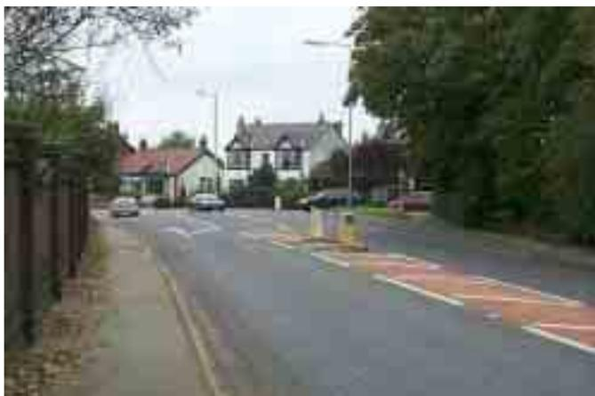
3.14 The overtaking deterrent effect of central hatching can be enhanced by the introduction of refuges either as a single feature or as a series along the road. The visibility of refuges should be emphasised by the installation of illuminated refuge indicator lamps. This is particularly important when refuges are installed on unlit roads where damage to the actual illuminated bollards may create visibility problems at night.
