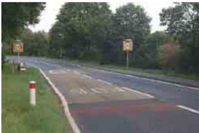
3.48 Changes in surface texture can be used on the approaches to hazards or gateways. Textured surfacing can provide a visual, audible and vibratory warning to drivers but to a lesser degree than rumble devices or rumble areas. It is important to ensure that skid resistance is maintained. This is best achieved through the use of a high skid resistant surfacing.
