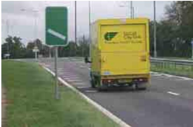
3.32 Countdown signs can be used to indicate the distance in hundreds of yards to a roundabout or the next point at which a driver may leave a route. Although mainly intended for roundabouts and non-lane drop grade separated junctions, they might also be appropriate at at-grade junctions where deceleration lanes are provided.
