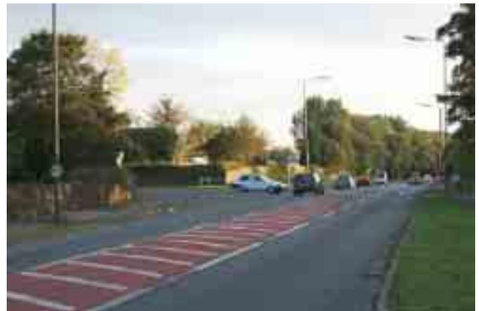
3.13 The virtual reduction of carriageway width by the use of central hatching is a common feature of trunk road traffic calming schemes. The hatching can be used to deter overtaking and can be widened to incorporate protected right turning facilities. Coloured surfacing is often used in conjunction with hatching to emphasise the presence of the markings. The impact on the character of the route and specific location should be considered. (See Section 3.16).
