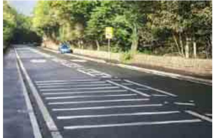
3.41 Rumble devices are designed to alert drivers to approaching hazards or gateways through noise, vibration and visual effect. Devices may be referred to as rumble bars, jiggle bars, rumble strips or rumble areas. Bars or strips are usually formed of thermoplastic and must not exceed 15mm in height and no vertical face may exceed 6mm in height. Adequate audible and vibratory warning can be achieved from 13mm high rumble devices.
