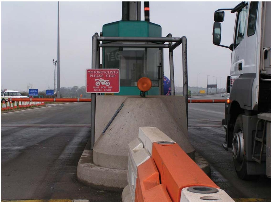
**Figure 3/4 Hazard Warning Beacons Fixed to Concrete Bollard**
