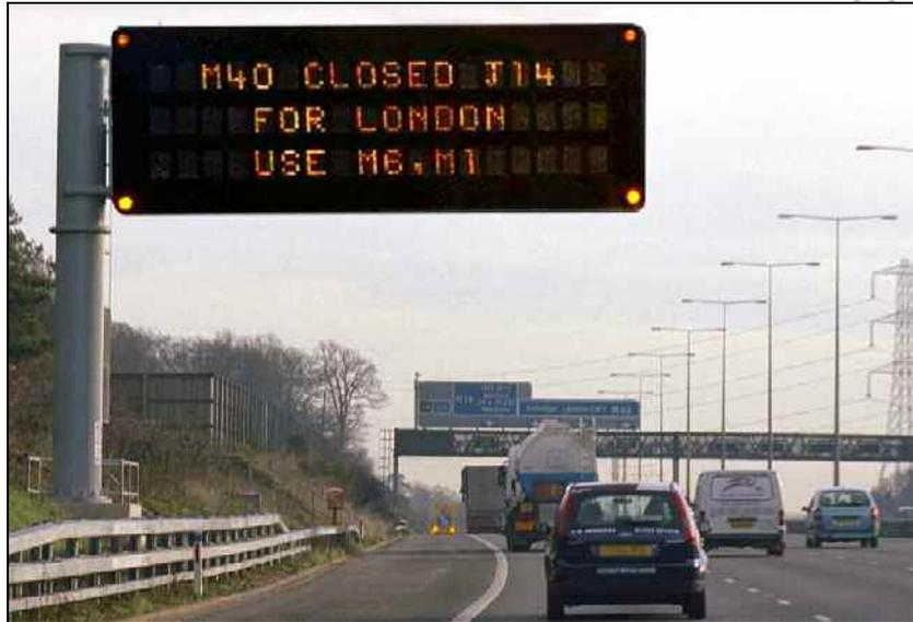
**Figure 3. 3 x 18 Motorway Signal Mark 3 (MS3)
