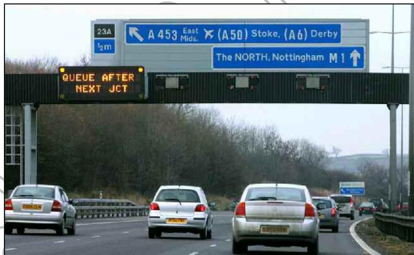
**Figure 5. Portal gantry mounted 2 x 12 Message Sign.**
