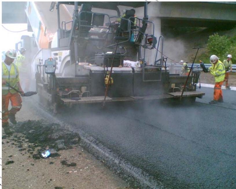
**Figure 6.1. The second of two paving machines laying the second rip of a TSCS so that both rips can be compacted simultaneously whilst hot.**
