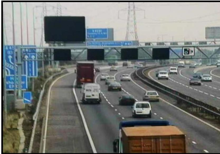
In normal state, MIDAS will operate at all times. MIDAS, if required, will set dynamic speed limits above all open traffic lanes (and a Red X if the hard shoulder is not open) as shown in the photograph below.
