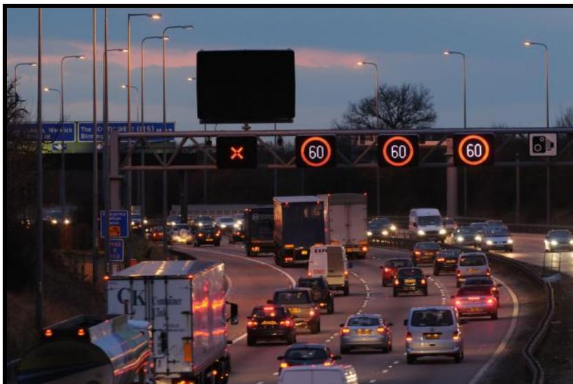
This will also be the mode of operation for any sections of controlled motorway. In controlled motorway schemes, there is a hard shoulder that is never used as a running lane, but gantries are installed according to advice given in IAN 111/09 so that VMSL can be used to control traffic on the main carriageway. In this case there will not be an AMI over the hard shoulder.
