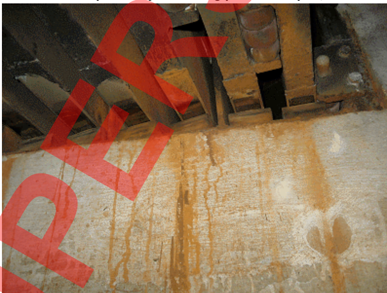
Figure E.5 Cable-stayed bridge (Composite steel-concrete deck) Built 1991 - Corrosion to expansion joint sliding plates over pier, circa 2007
