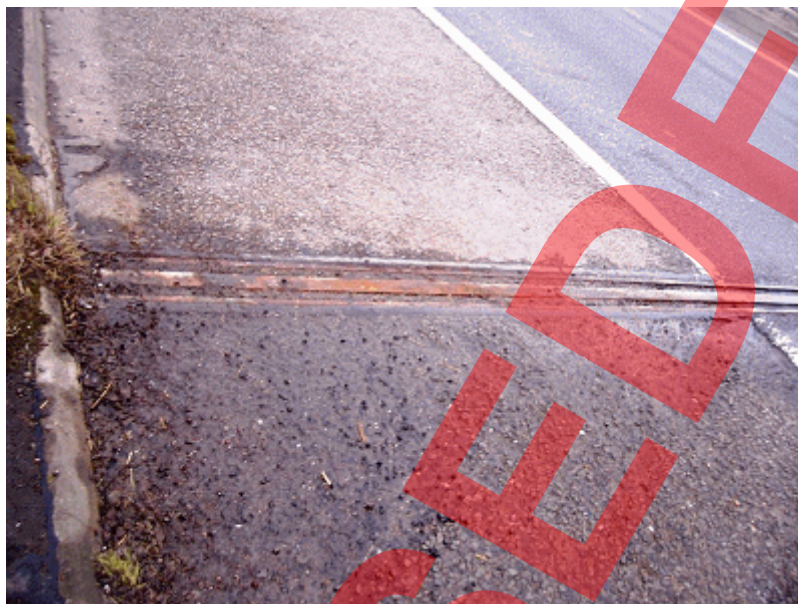
Figure E.9 Viaduct (in-situ pre-stressed concrete). Built 1990 - Corrosion to rails and debris in seals
