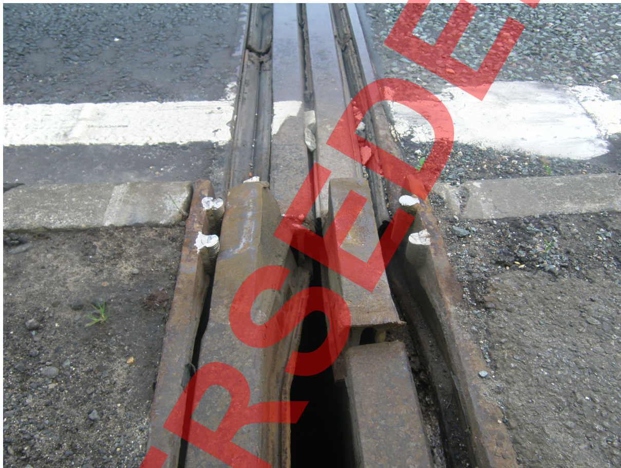
Figure E.6 Viaduct (Pre-cast pre-stressed concrete) Built 1976- Failure of joint footway. Seal failed between rails on carriageway
