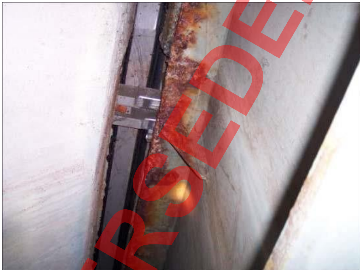
Figure E.8 Viaduct (in-situ concrete deck). Built 1986 - Damage to the west deck expansion joint - rail broken in the middle and level difference in carriageway surface
