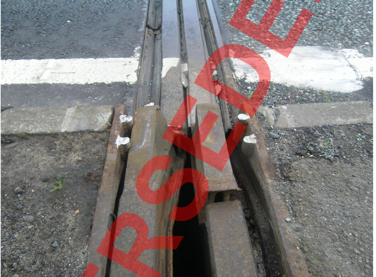
**Figure E.7 - Cable-stayed Bridge (composite steel-concrete deck). Built 1991 - Trimmer beam support steelwork corroded.**
