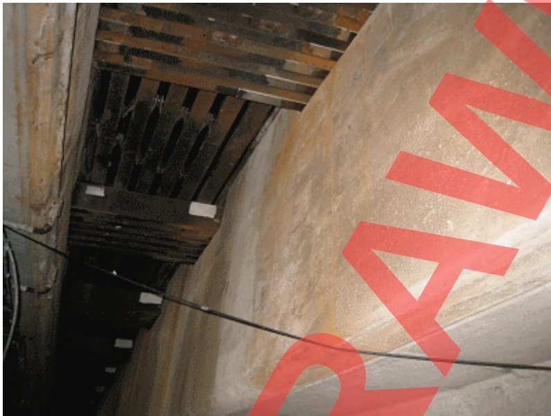
Figure E.4 Cable-stayed bridge (composite steel-concrete deck) Built 1991 - Rust staining from expansion joint over pier (Seal replacement stopped water ingress, circa 2007)
