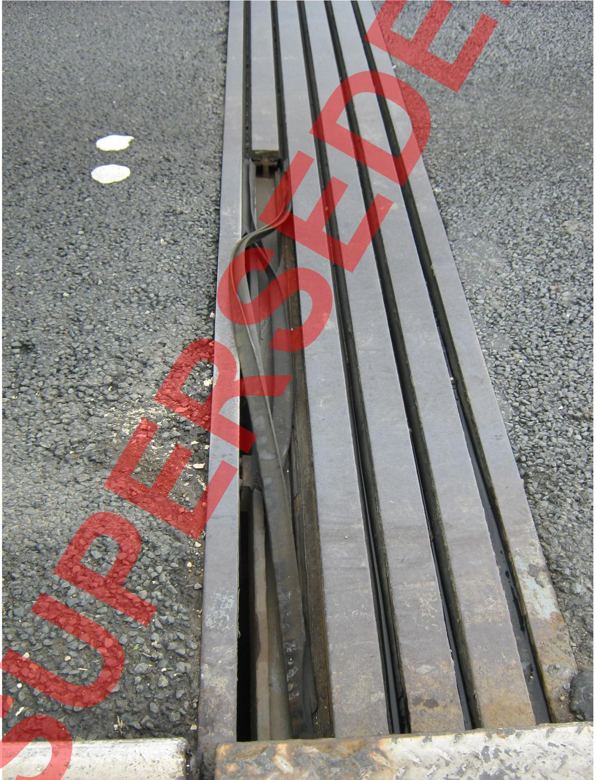
A full internal inspection of the abutment was arranged, which revealed extensive damage to the joints,
