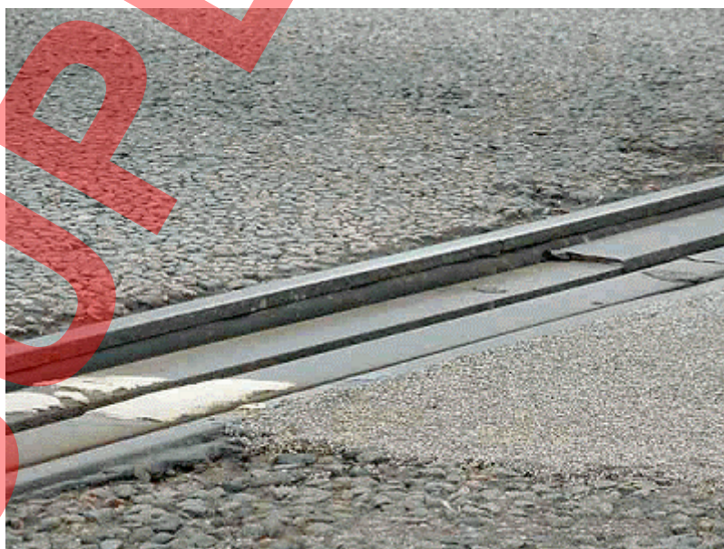
Figure E.8 Viaduct (in-situ concrete deck). Built 1986 - Damage to the west deck expansion joint - rail broken in the middle and level difference in carriageway surface
