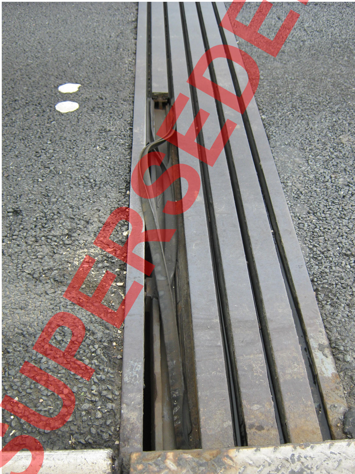
Figure E.2 Viaduct (precast prestressed concrete) built in 1993- The damaged rail has been taken out of the joint and corrosion is visible on the rails
