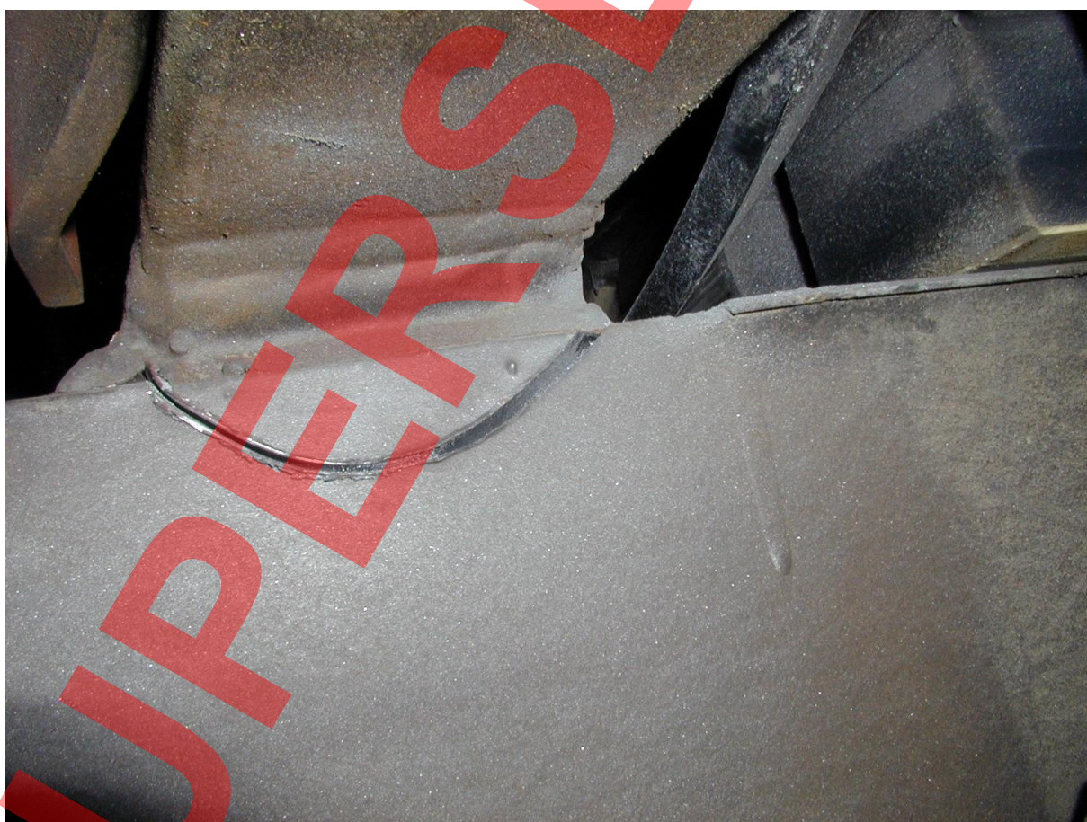
Figure E.3 Cable-stayed bridge (composite steel-concrete deck) Built 1991 - Fracture in the support joist immediately below the welded connection to the rail
