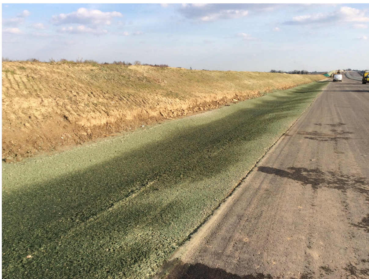
Figure 3.29.1 Example of hydro-seeded trapezoidal grassed surface water channel shortly after construction (Photo courtesy of Norfolk County Council & Balfour Beatty)
