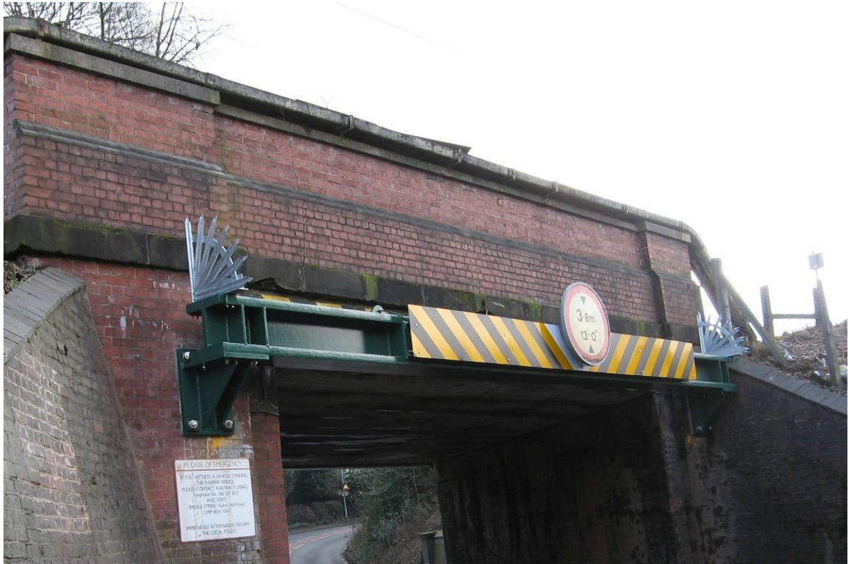
Figure A.5 Collision protection beam to flat soffit bridge supported from abutment Cills
