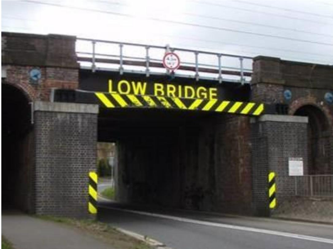
Figure A.7 Collision protection beam to arch at height of chord markers
