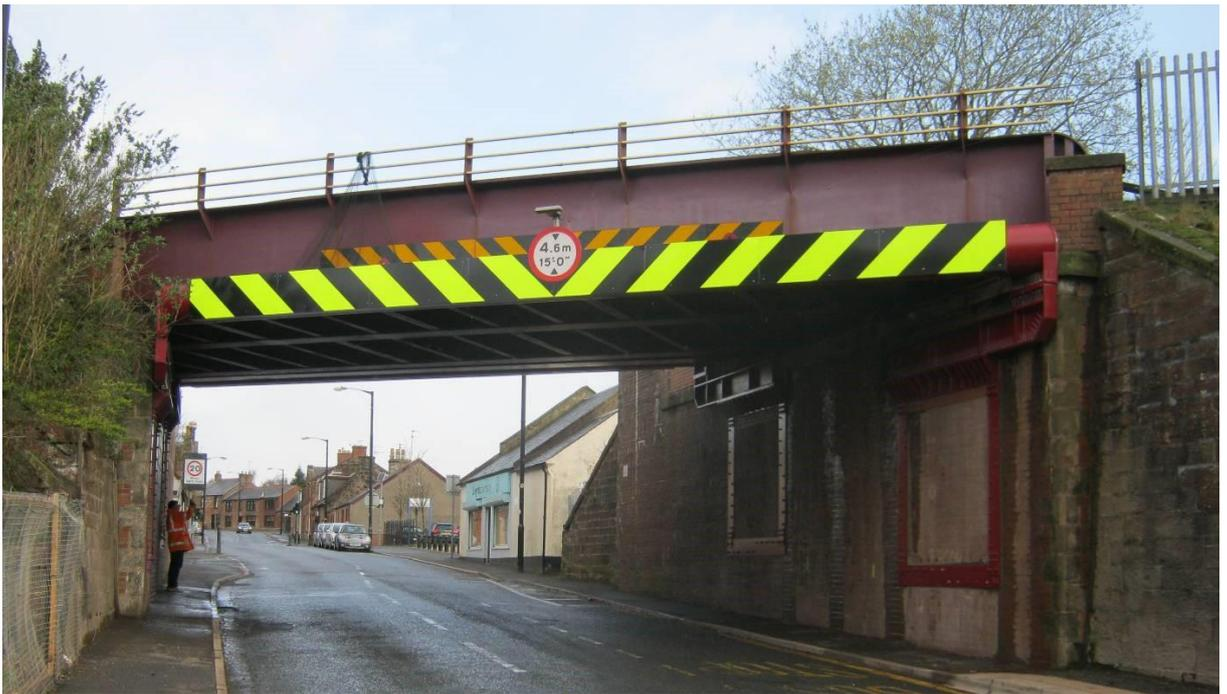
Figure A.2 Collision protection beam abutment supports
