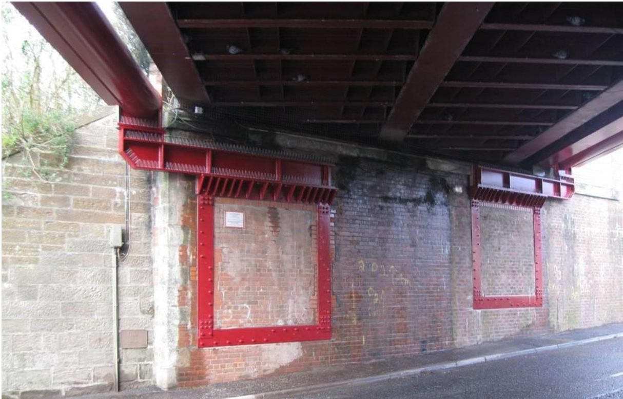
Figure A.2 Collision protection beam abutment supports
