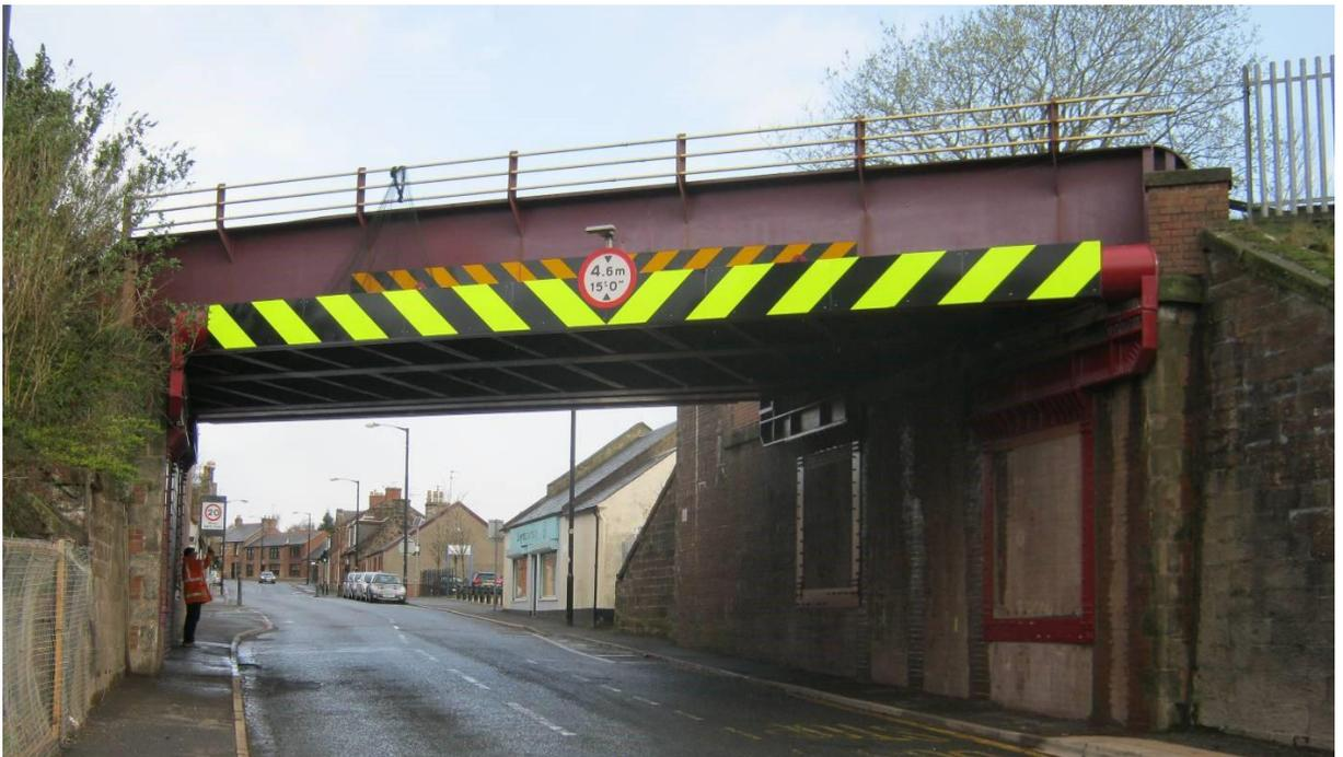
Figure A.2 Collision protection beam abutment supports
