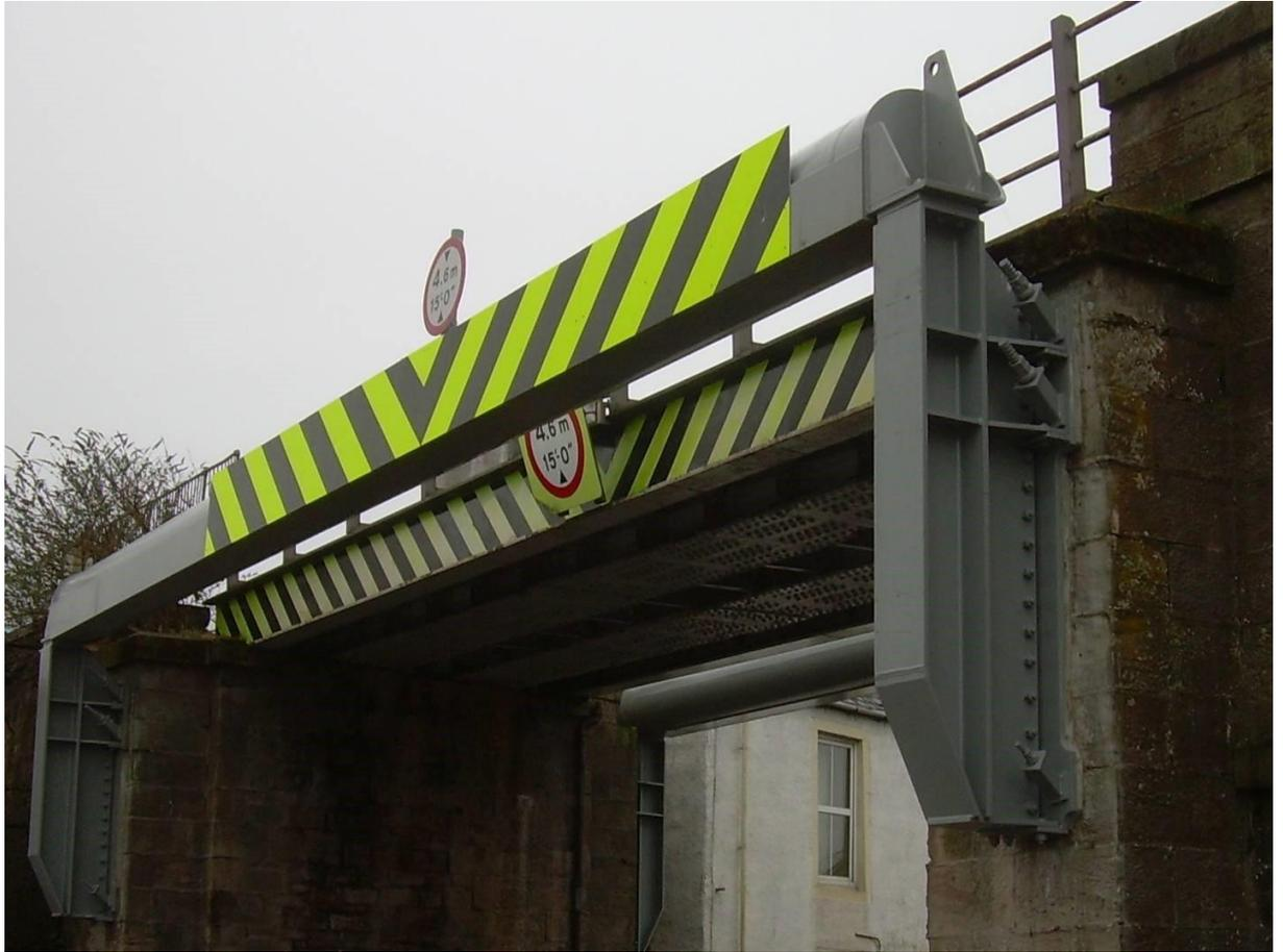
Figure A.4 'I' shape collision protection beam with chevaux de frise
