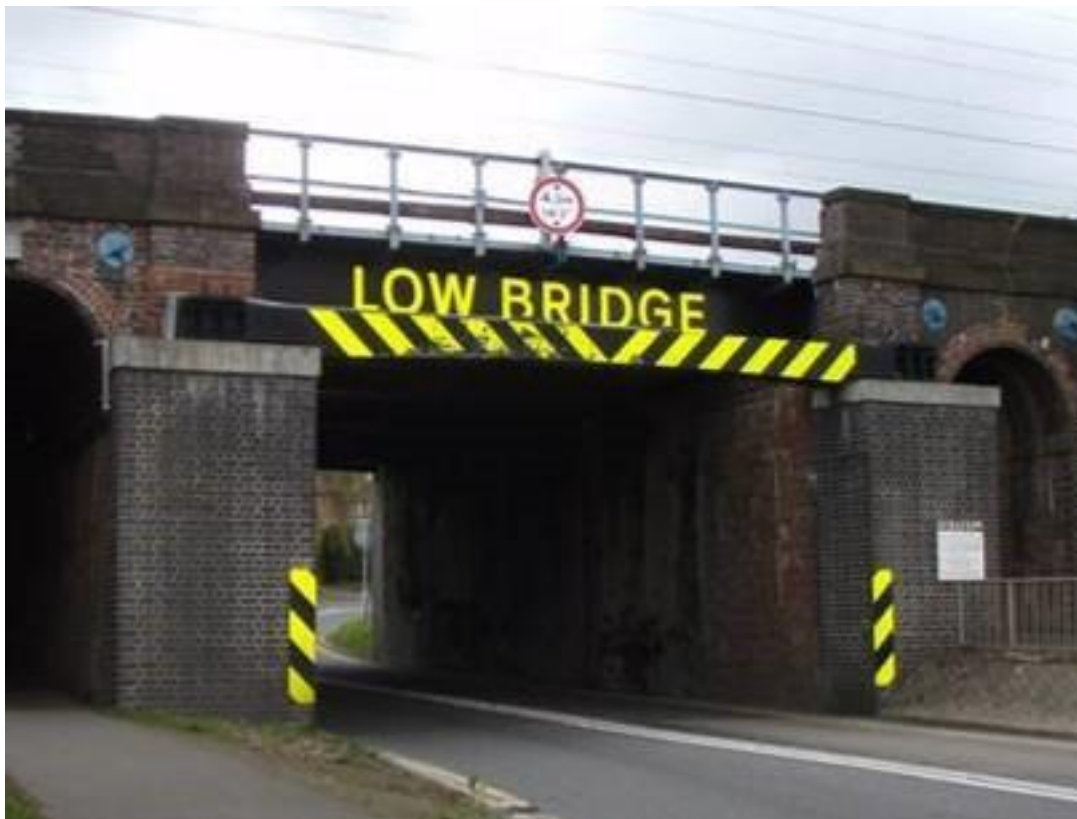
Figure A.6 Collision protection beam to flat soffit bridge supported from abutment extensions. Note the camber to the beam
