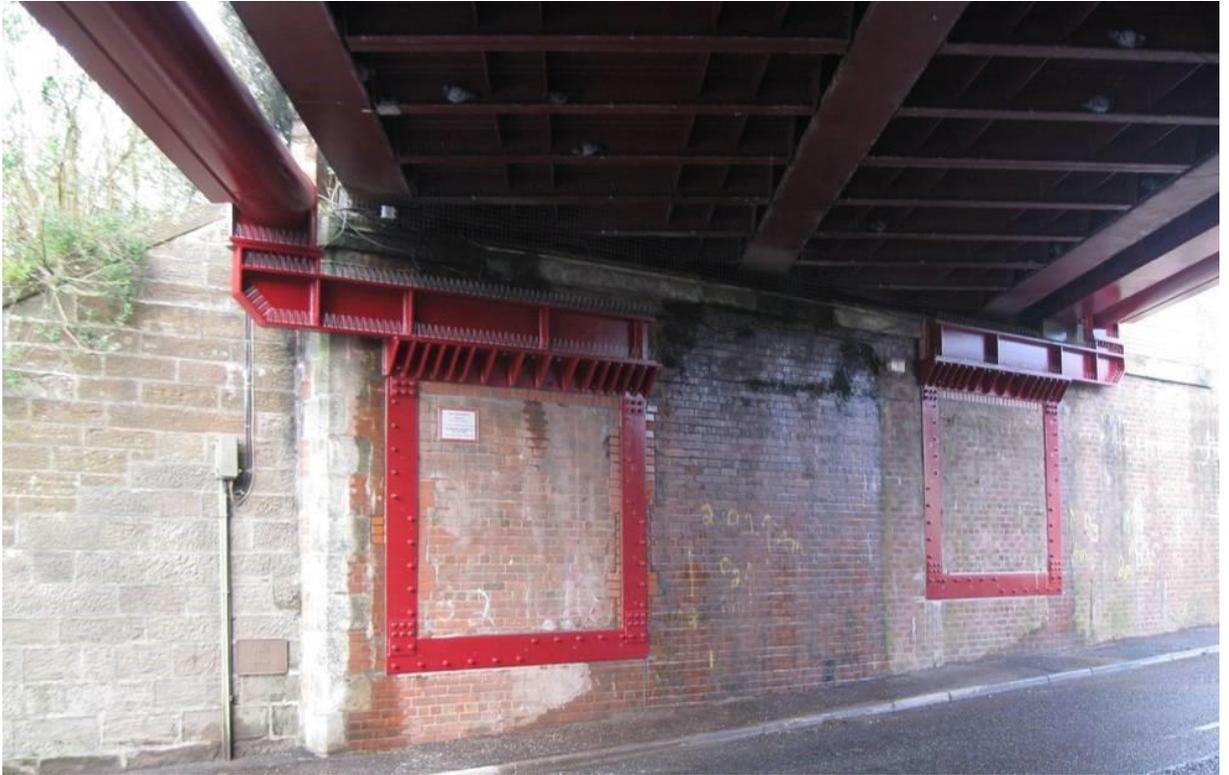
**Figure A.3 Circular collision protection beam to flat soffit bridge showing abutment supports**
