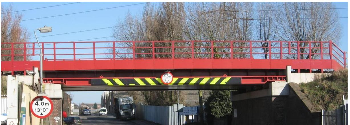
**Figure A.6 Collision protection beam to flat soffit bridge supported from abutment extensions. Note the camber to the beam**
