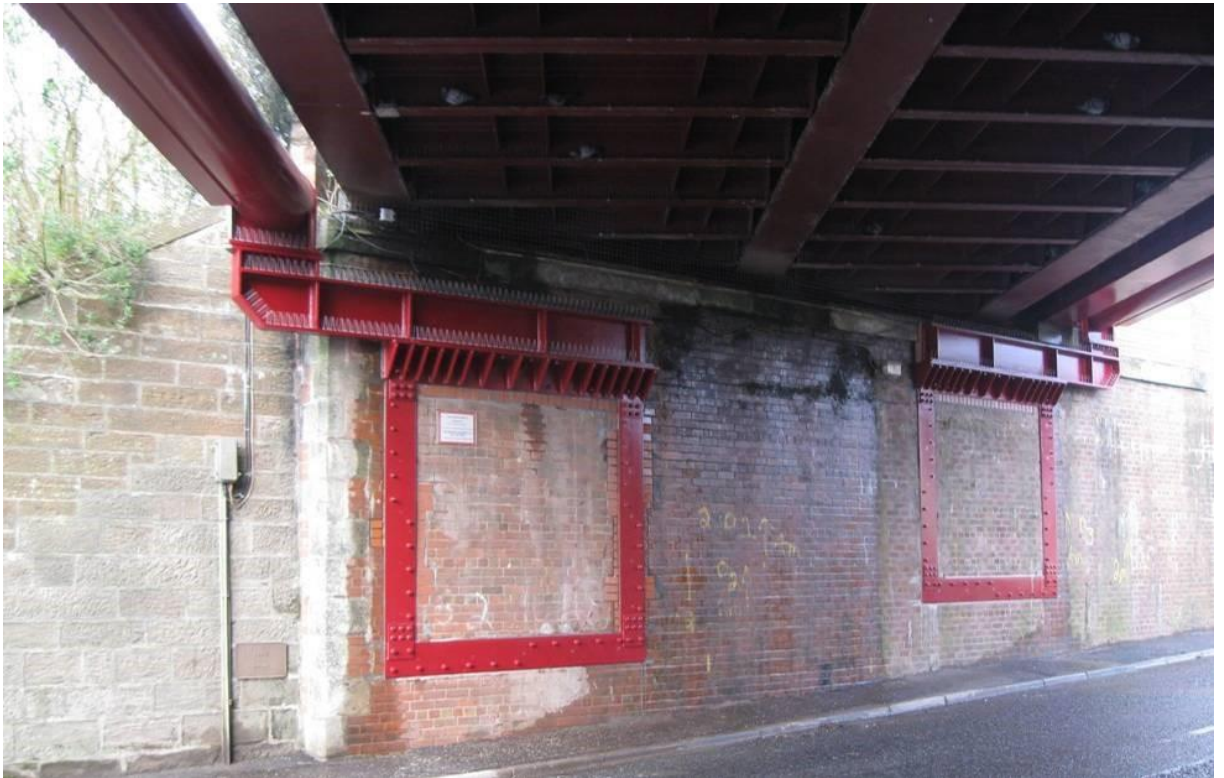
Figure A.2 Collision protection beam abutment supports
