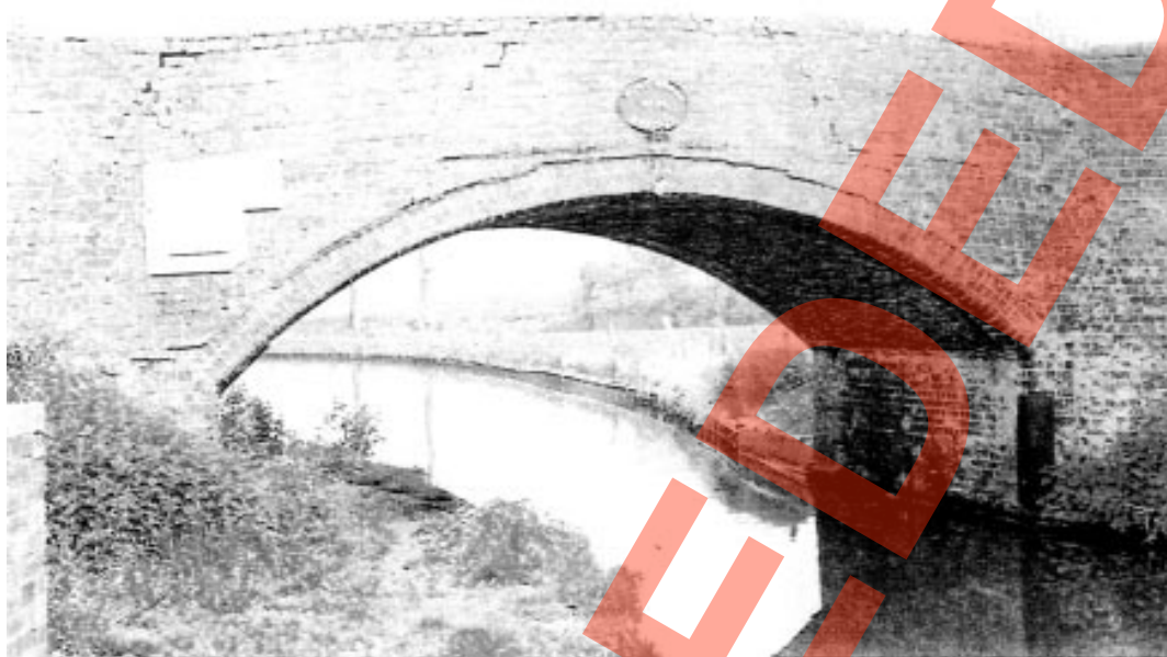
Plate 11 This shows cracking of the spandrel/parapet walls which suggest a flexible arch barrel.
