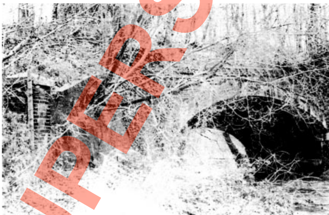
Plate 12 This shows vegetation growing from the faces of the bridge and wing walls; this vegetation should be cut back before it has a chance to damage the brickwork.
