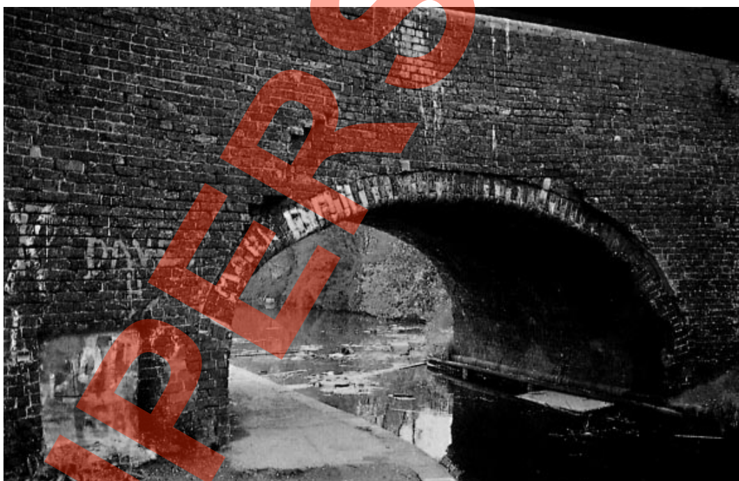
Plate 9 This illustrates the movement of spandrel walls.
