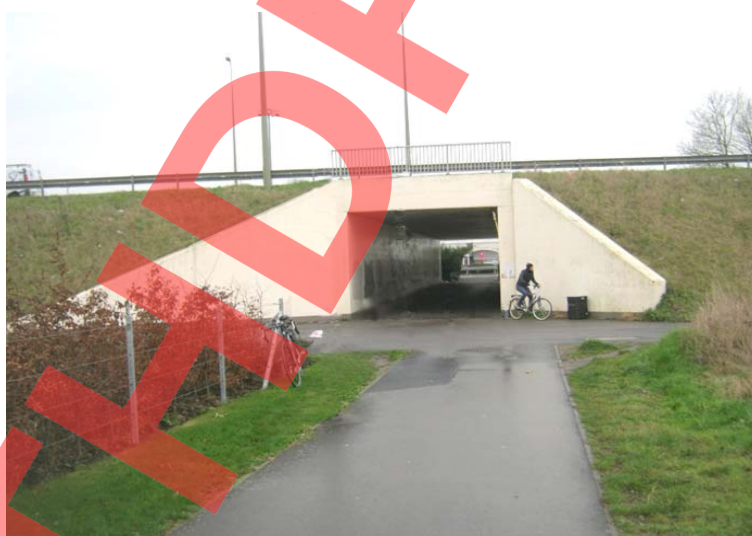
Figure 2.5.2 Straight Approaches, Wide Profile and Flared Wing Walls Help to Maximise Visibility
