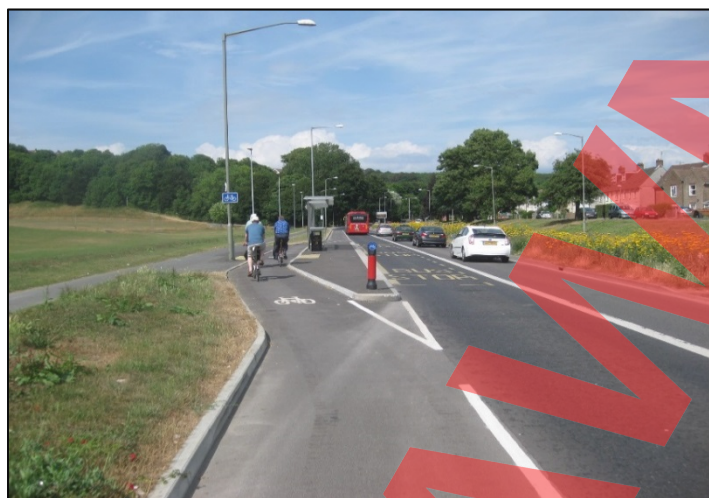
Figure 2.3.6 Cycle Lane with Bus Stop Bypass
