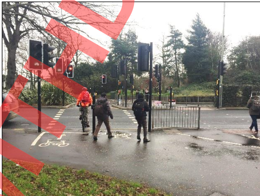
Figure 2.4.8.1 Angled crossing (may be used where central refuge cannot accommodate a full stagger)
