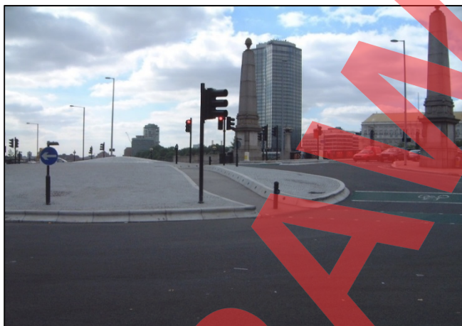
Figure 2.7.3 Cycle Track across the Central Island of a Signalised Roundabout
