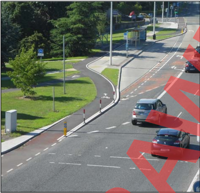
Figure 2.3.9.1 Cycle Lane merges into Cycle Track (not UK)
