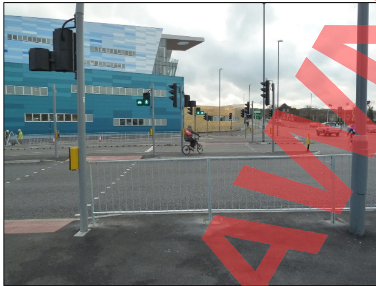
Figure 2.4.8 Staggered crossing (only to be used where central refuge can accommodate the design cycle and cycle track parameters)
