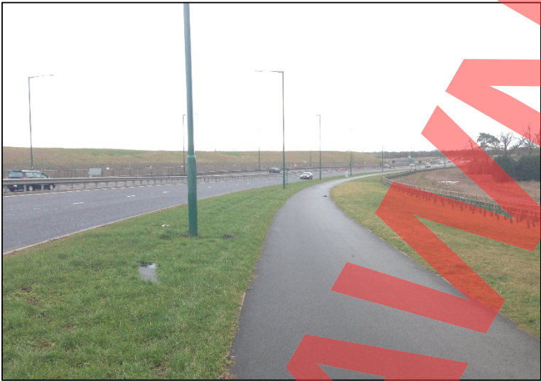
Figure 2.3.2.5 Cycle Track with Wide Verge
