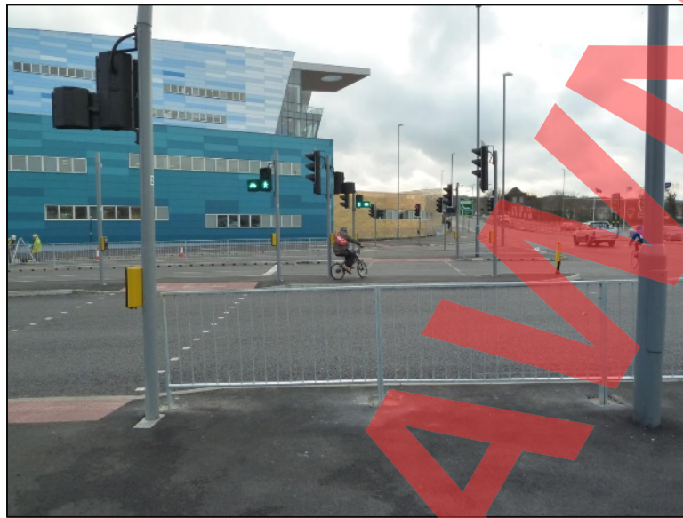
Figure 2.4.8 Staggered crossing (only to be used where central refuge can accommodate the design cycle and cycle track parameters)
