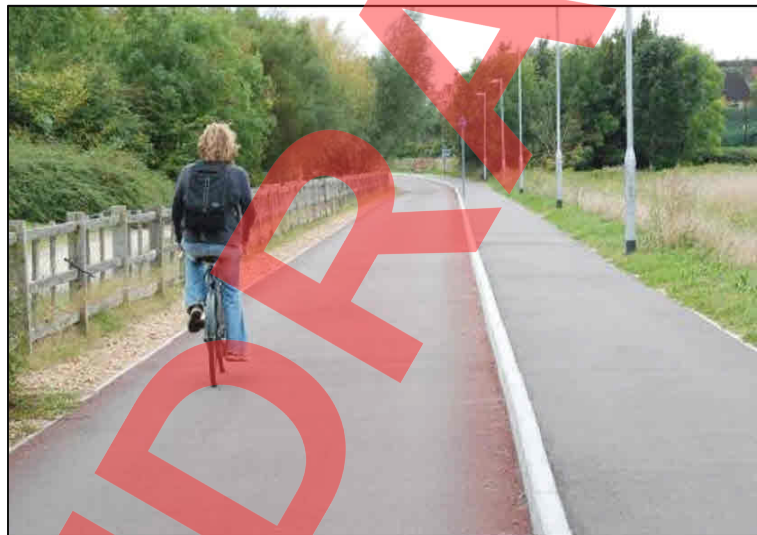
Figure 2.3.2.2 Cycle track and Footway Separated by Level with Good Quality Surface and Lighting
