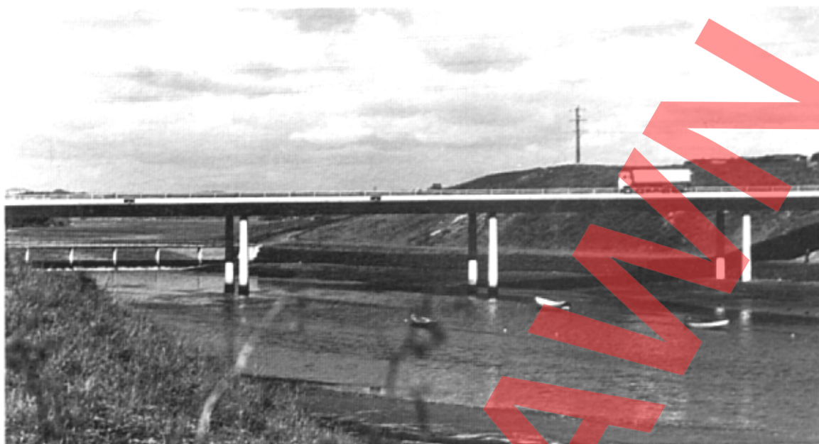
Figure 6. The effect of a light fascia over beams shaded by a substantial cantilever. This is less marked when the sky is overcast.
