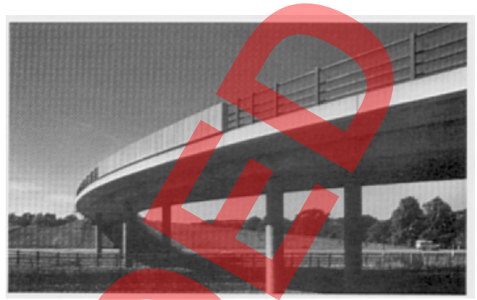
Figure 12. Treatment of a high containment parapet to emphasise the continuity of the deck. A step in the face of the parapet to create a shadow line, and a different surface, which should not be overdone.
