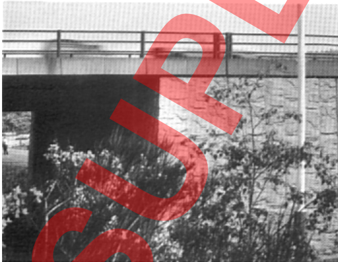
Figure 16a. Ribbed and moulded surfaces in a very dirty atmosphere. Nine years after completion. The mark on the fascia to the left is the shadow of the post. The whole surface is extremely dirty, but uniformly so.
