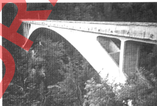
Figure 7. The scuppers in the parapet of the Salginatobel Bridge are there to allow water from the deck to drain away. They also add interest to the bridge when seen close to, and reduce the apparent scale. There may be more scuppers than function strictly requires.
