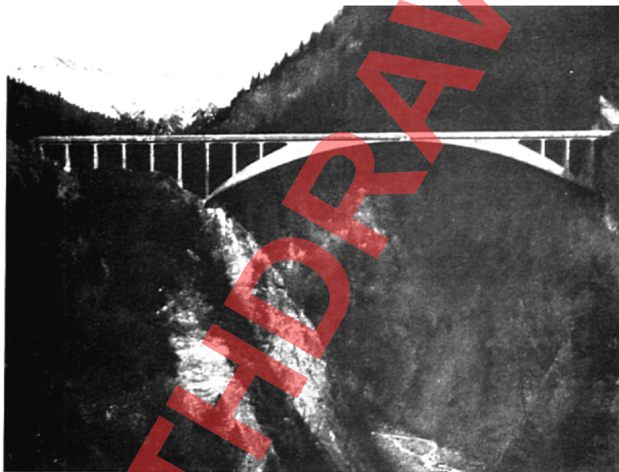
Figure 3a. Maillart's Salginatobel Bridge is extremely simple and produced the lowest tender in a design/construct competition.
