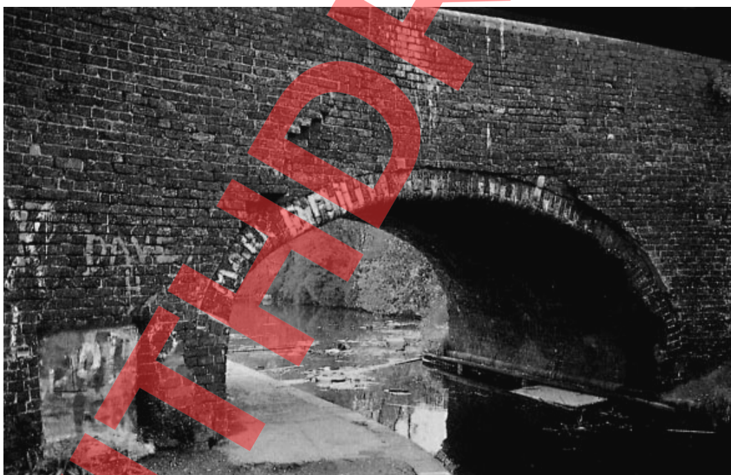
Plate 9 This illustrates the movement of spandrel walls.
