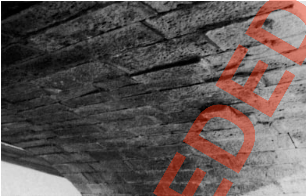
Plate 8 This illustrates the radial displacement of individual stones. In this particular case the assumed thickness of the arch barrel was adjusted to take account of the displacement.
