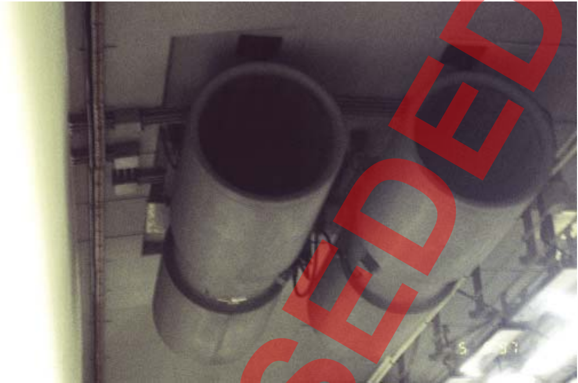
Figure 7.1: Jet Fans providing Longitudinal Ventilation
